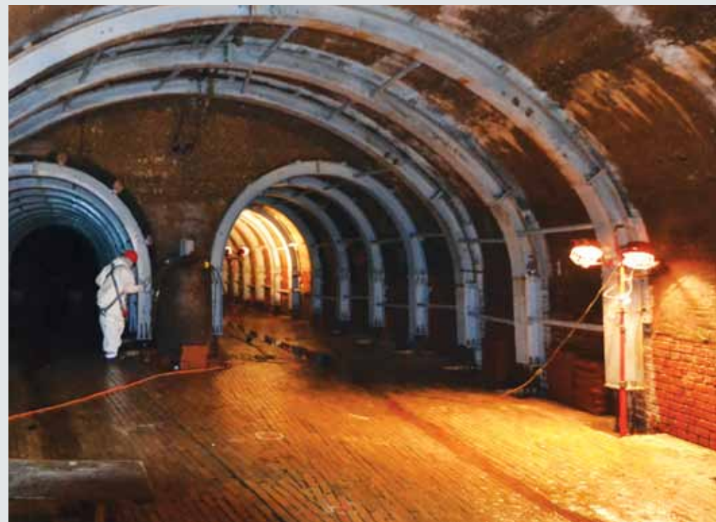
Near right: To prepare for the DC Clean Rivers Project tunnel system running underneath it, the Tiber Creek Sewer got arch support from the installation of these steel ribs.
