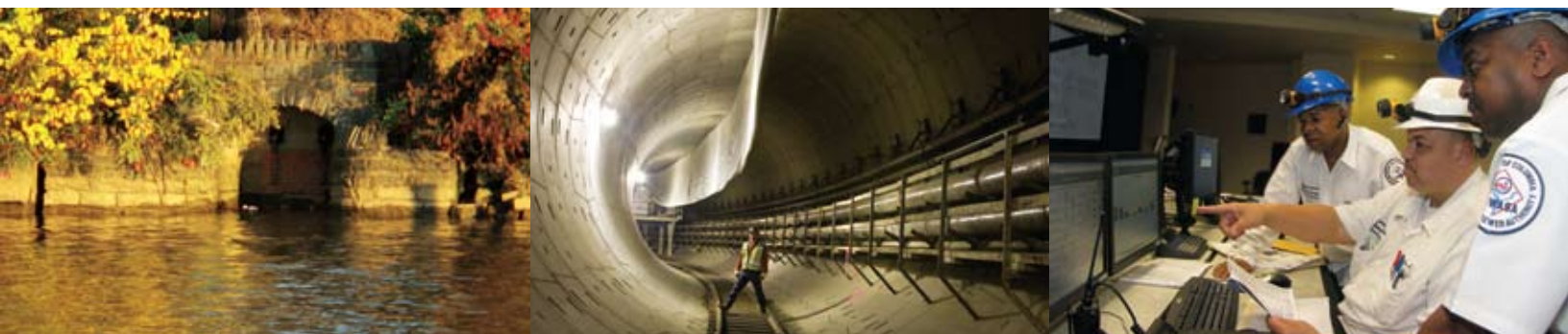
LEFT: In wet weather, CSOs can enter waterways from outfalls like this one.
