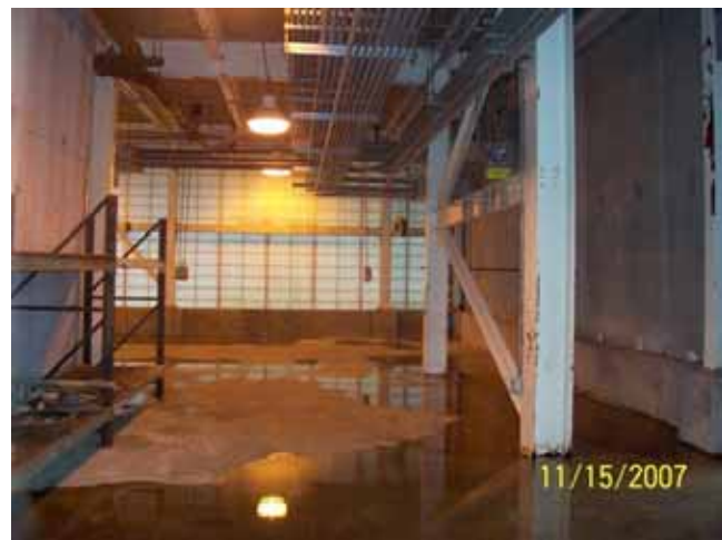
(Left): When biosolids conveyors were hosed with water, dirty water flowed through openings in the floor to lower level storage wells and areas used for equipment storage, shown here. (Right): Good housekeeping practices eliminated the need for water, and here, the equipment storage area is shown after it was cleaned up – and could remain that way.
