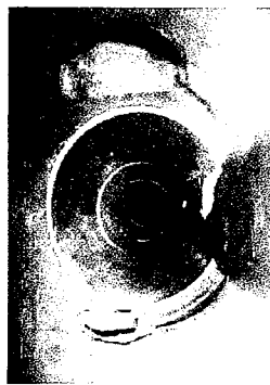
Date: 08/29/2006 Dist: 34.3 Ft Obs: Tap Factory Active
