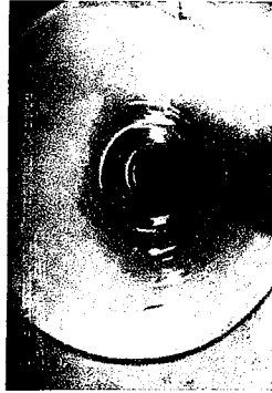
Date: 08/29/2006 Dist: 89.7 Ft Obs: Deposits Attached Grease
