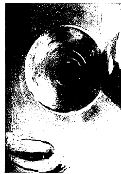
Date: 08/29/2006 Dist: 71.5 Ft Obs: Tap Break-in Intruding
