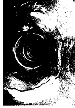
Date: 08/29/2006 Dist: 171.0 Ft Obs: Deposits Attached Grease
