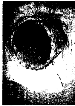
Date: 08/29/2006 Dist: 25.1 Ft Obs: Tap Break-in Active
