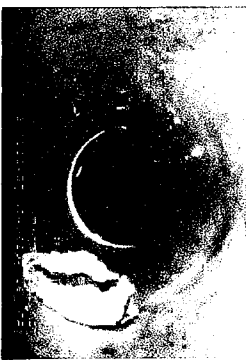
Date: 08/01/2006 Dist: 129.2 Ft Obs: Tap Break-in Defective
