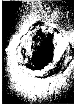
Date: 08/29/2006 Dist: 127.7 Ft Obs: Tap Break-in Active
