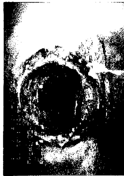
Date: 08/29/2006 Dist: 55.6 Ft Obs: Tap Break-in Active
