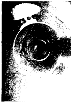
Date: 08/29/2006 Dist: 20.1 Ft Obs: Tap Factory Active
