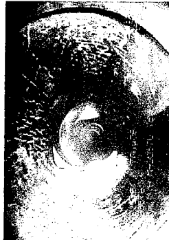
Date: 08/29/2006 Dist: 215.6 Ft Obs: Crack Multiple
