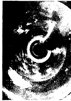
Date: 08/29/2006 Dist: 101.3 Ft Obs: Hole
