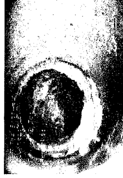
Date: 08/29/2006 Dist: 18.7 Ft Obs: Tap Break-in Active
