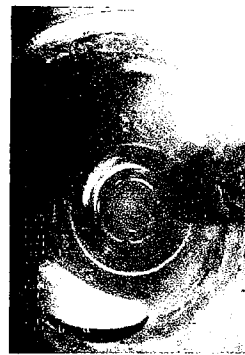
Date: 08/29/2006 Dist: 89.7 Ft Obs: Deposits Attached Grease
