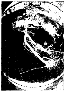
Date: 08/01/2006 Dist: 153.8 Ft Obs: Roots Tap Connection
