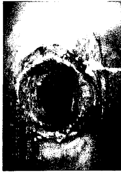
Date: 08/29/2006 Dist: 55.6 Ft Obs: Tap Break-in Active
