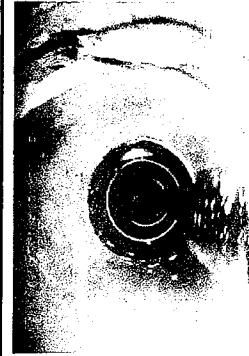
Date: 08/29/2006 Dist: 16.7 Ft Obs: Tap Break-in Active
