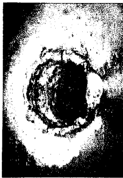
Date: 08/29/2006 Dist: 79.8 Ft Obs: Tap Break-in Active
