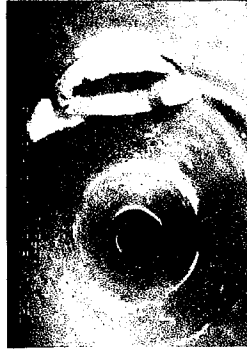
Date: 08/29/2006 Dist: 62.1 Ft Obs: Tap Break-in Defective
