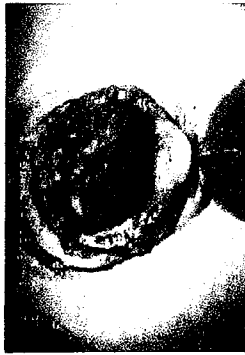
Date: 08/29/2006 Dist: 202.4 Ft Obs: Tap Break-in Active
