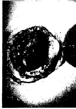
Date: 08/29/2006 Dist: 202.4 Ft Obs: Tap Break-in Active
