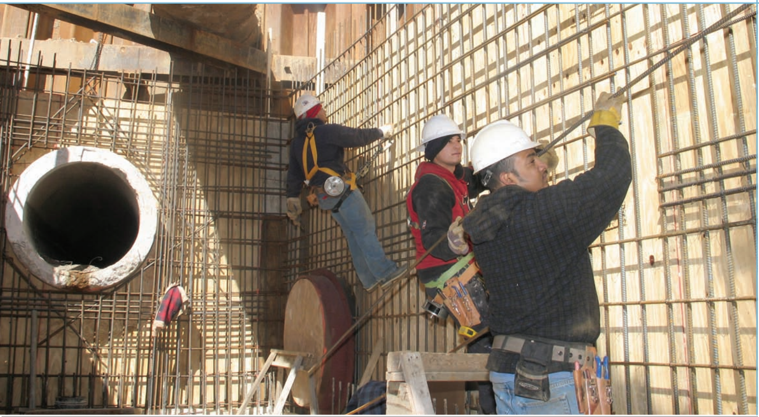
Men at work on the junction chamber of the new Eastside Pumping Station . The pipe shown connects to the sewer bringing wastewater into the chamber before it is pumped to Blue Plains.
