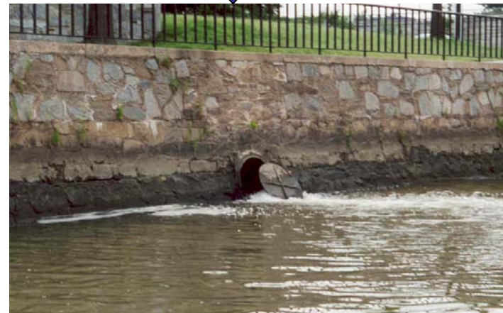
Discharges to River
