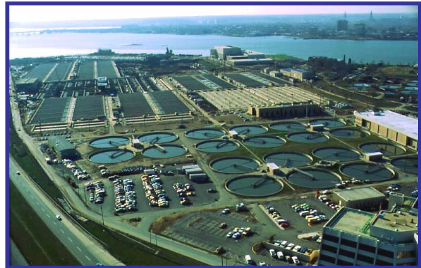
Blue Plains Wastewater Treatment Plant
