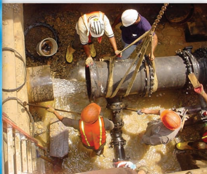
The replacement and rehabilitation of water mains and valves is a major priority in WASA's water quality improvement program.
