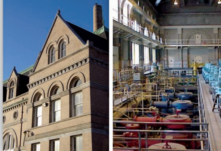
Major renovations at the Bryant Street Pumping Station include new high lift pumps, HVAC upgrades, and architectural improvements to the 100-year-old building.
