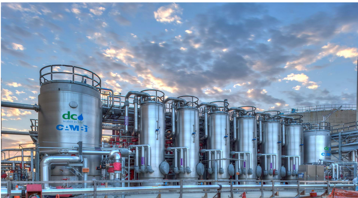
The Cambi Thermal Hydrolysis Process (THP) at the Blue Plains Advanced Wastewater Treatment Plant
