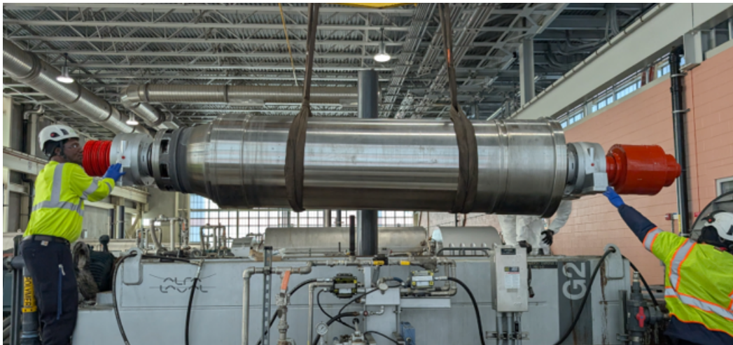
The picture shows DC Water staff aligning a large stainless-steel mechanical component part of wastewater treatment solids-processing equipment inside a maintenance facility. This highlights the heavy-duty equipment and precision mechanical work required to maintain DC Water's process engineering operations
