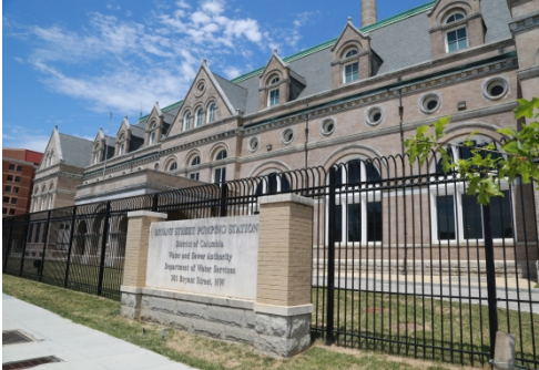
Bryant Street Pumping Station
