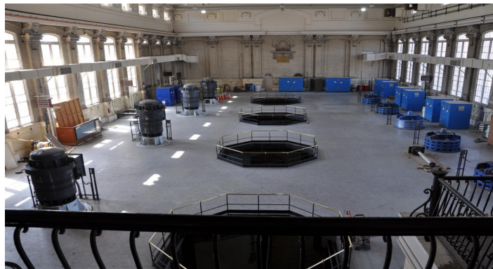
O Street Pumping Station
