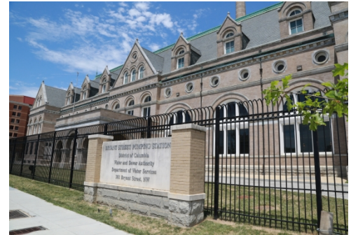
Bryant Street Pumping Station
