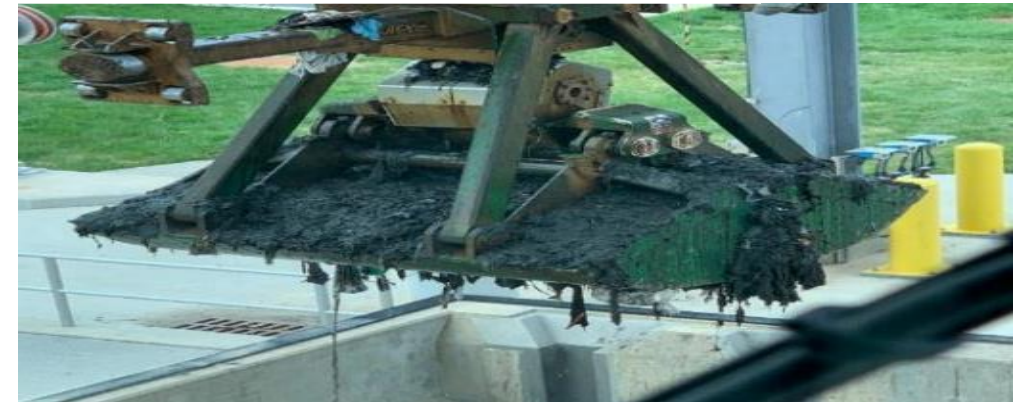
Trash, Debris and Solids Removal from Screening Shaft at Tunnel Dewatering Pumping Station
