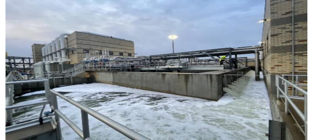
Enhanced Clarification at the Wet Weather Treatment Facility
