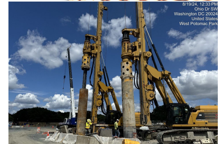
DCCR Potomac Tunnel Mining Shaft Construction
