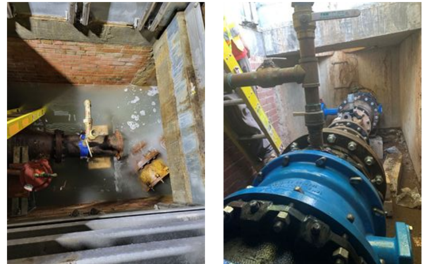
Water intrusion and repair photos at meter within vault
