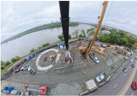
View of CSO 022 Construction Site and Shaft in August 2025
