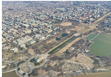
View of West Potomac Park Construction Site in February 2025
