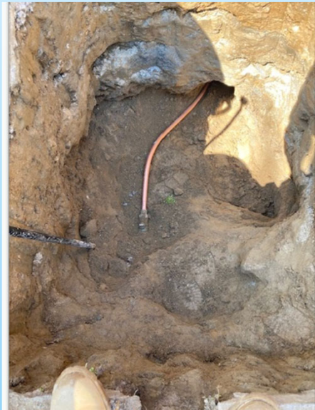
Excavated line at curb stop showing replaced pipe material
