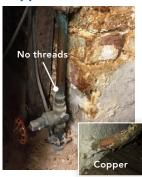
No "threads" on copper pipes. Green color is copper corrosion.
