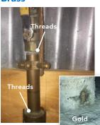
Brass pipes can have "threads."
