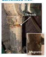
Galvanized pipes have "threads" at connections.
