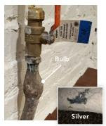
Lead pipes widen at base and often form a "bulb."
