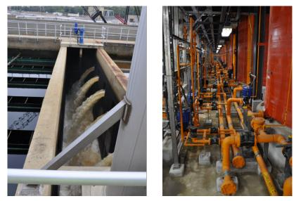
The left side picture shows a multimedia filter in backwash, flushing out contaminants. On the right, large tanks store ferric chloride, a key treatment chemical. This contrast highlights wastewater treatment operations
