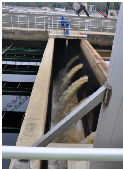
The left side picture shows a multimedia filter in backwash, flushing out contaminants. On the right, large tanks store ferric chloride, a key treatment chemical. This contrast highlights wastewater treatment operations
