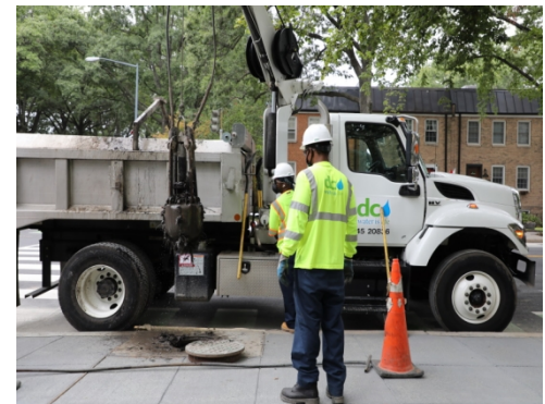
Sewer Inspection Maintenance Catch Basin
