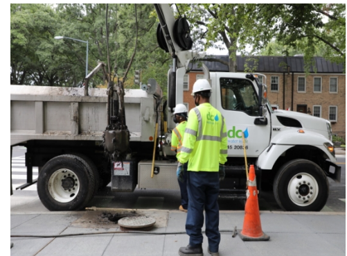
Sewer Inspection Maintenance Catch Basin
