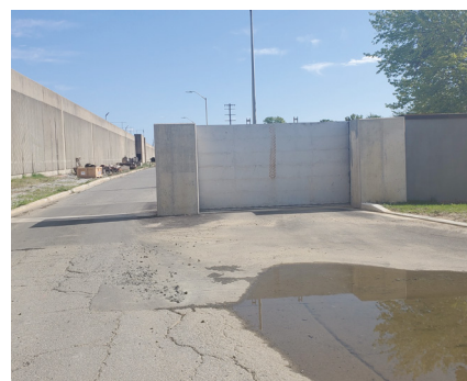
Blue Plains floodwall.
