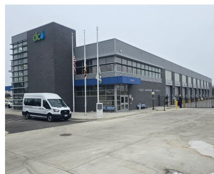
Fleet maintenance facility.
