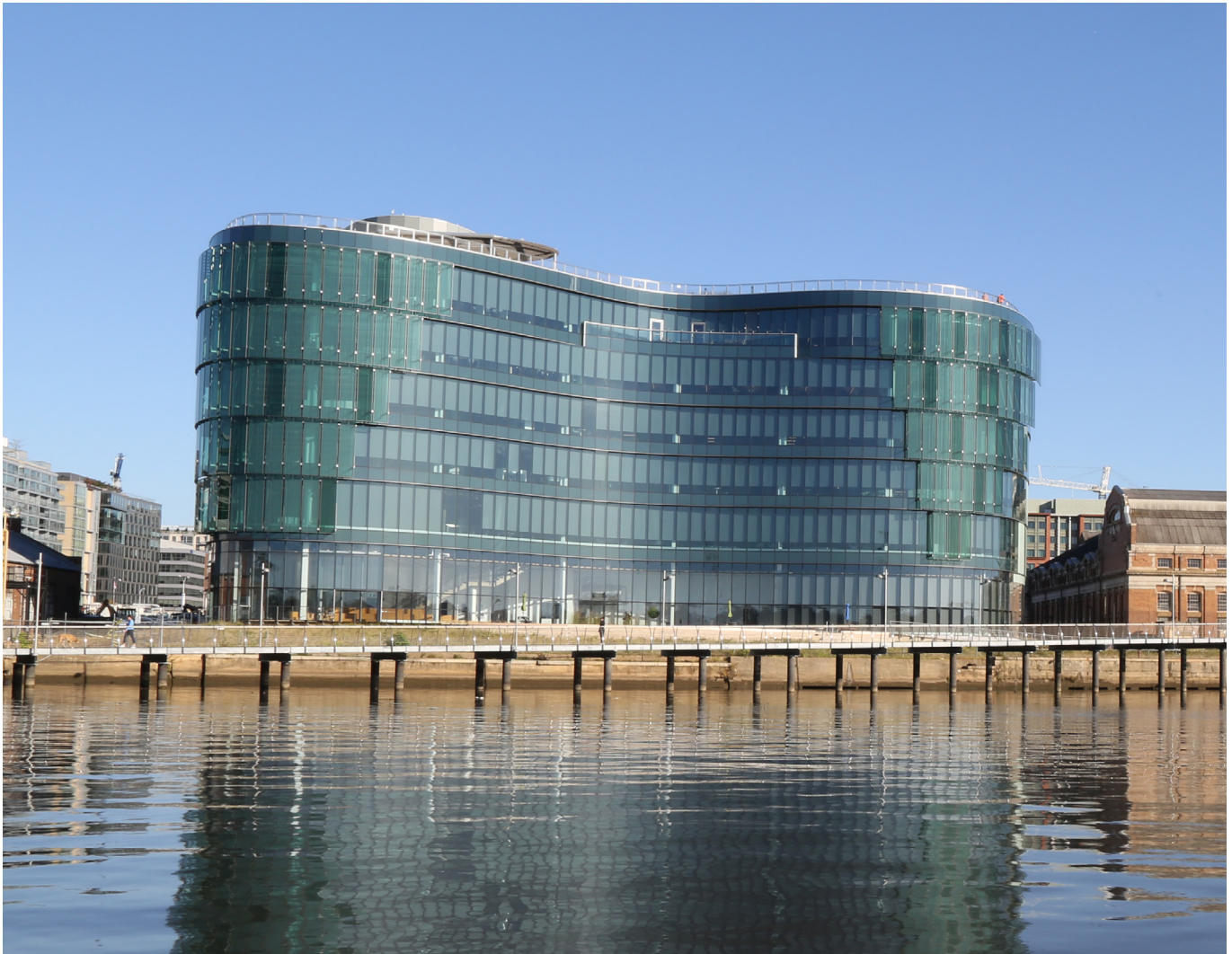
HQO, the headquarters for DC Water.
