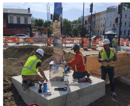
Contractors installing a sculpture at Cooper Gordon Park.
