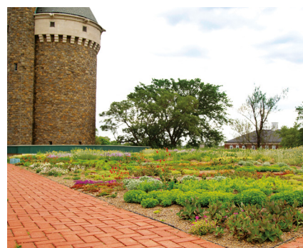
Green roof bioretention site at Fort Reno.
