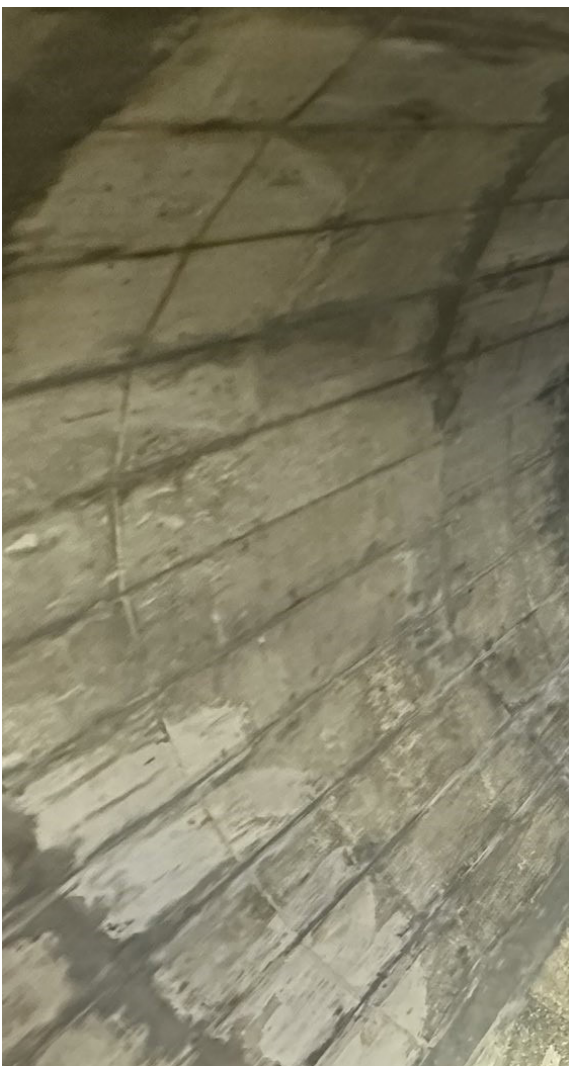
View of Northeast Boundary Tunnel shaft.
