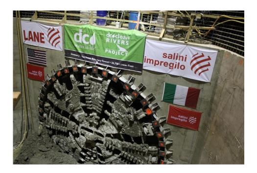
Chris, the Tunnel Boring Machine, broke through a wall of concrete to reach the W Street shaft, a key milestone in the mining of the Northeast Boundary Tunnel (NEBT). Chris rested for a bit in the shaft and received much-needed maintenance but is back underway now.
