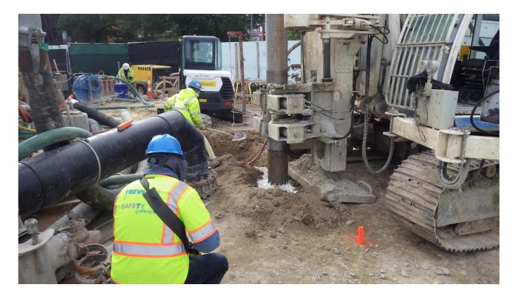
**Current Activity: Jet Grouting** The contractor will install jet grout columns on the north side of the intersection at First Street and Rhode Island Avenue NW. This is a process of injecting the soil with a cement to stabilize the soil. This work will continue to the end of August 2020.
