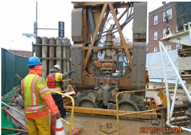
*Above: Workers guide the hydro-mill into the ground to begin construction of the drop shaft. Below: Pre-trench work at excavation site for the drop shaft.*
