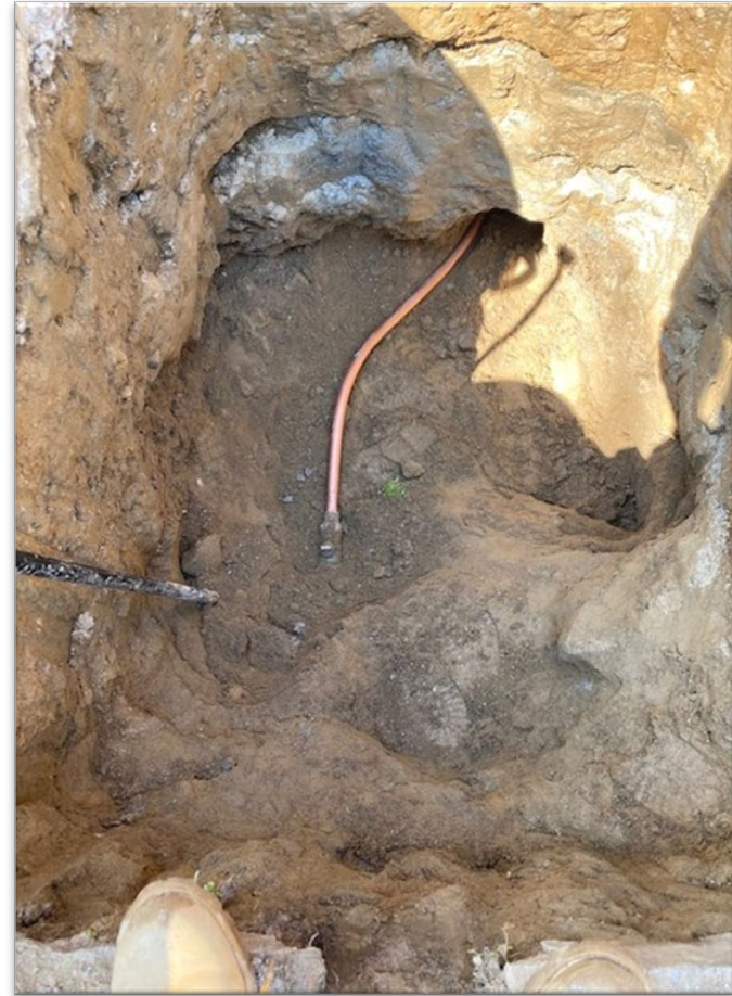
✓ Clear Copper Curb Stop Connection
