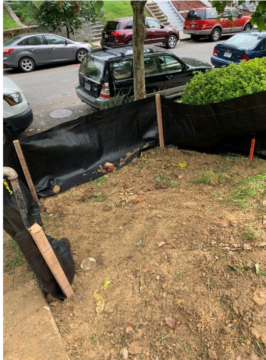
✓ Good Backfill
