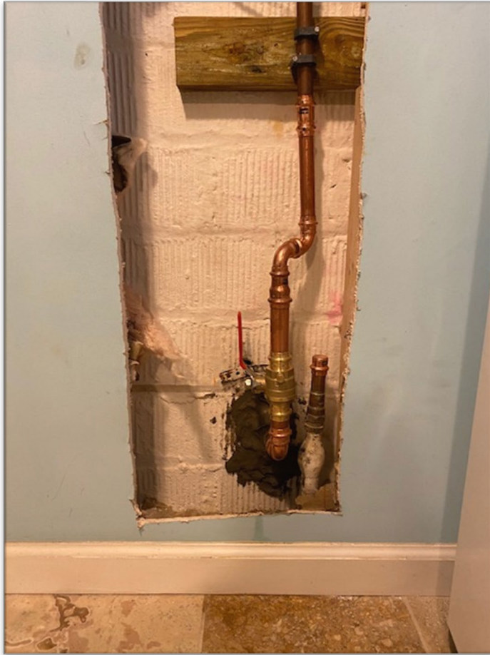
✓ Clear Copper First Fitting
