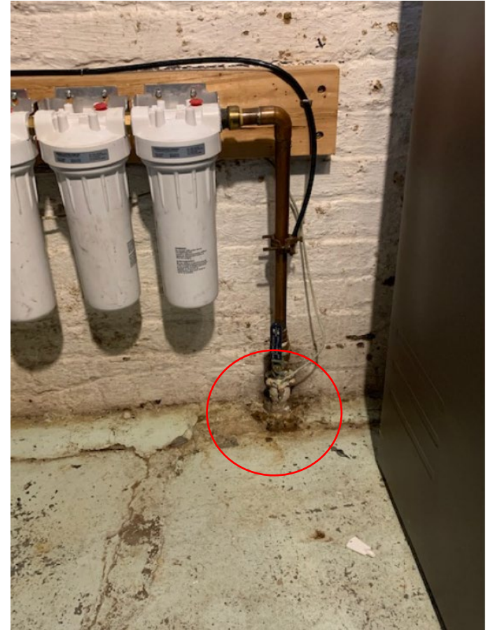
✓ Good 1 st Fitting Pic Breaking through Floor
