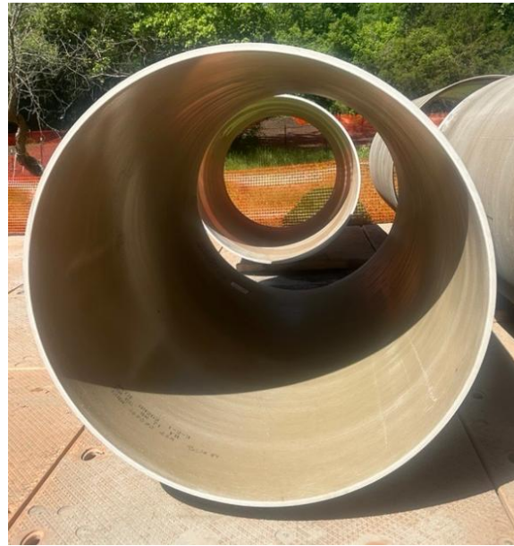
(Photo 2): Shows a typical 51-inch fiberglass reinforced pipe that will be used to slipline this section of the Potomac Interceptor.
