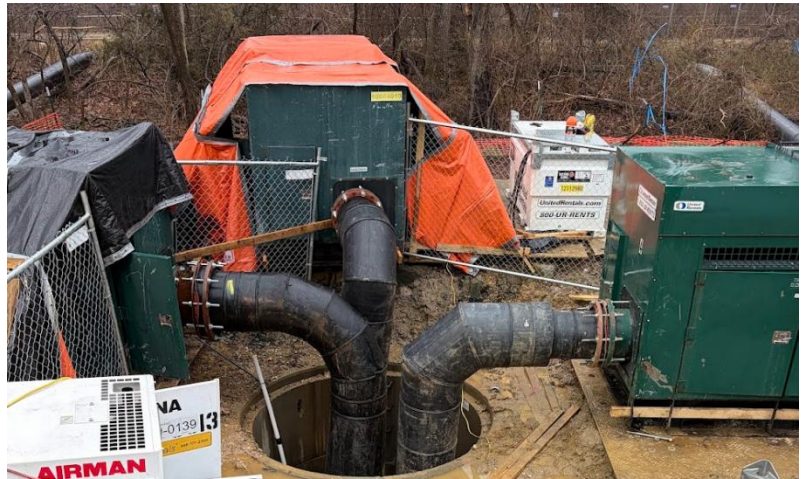
(Photo 2): Shows a typical bypassing pumping system. Pumping the wastewater out from a location and diverting it to a location around the work area.
