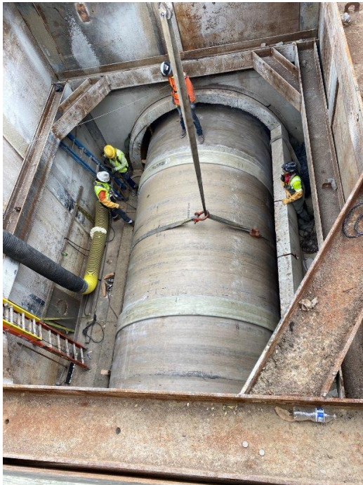
(Photo 1): Shows a typical launch and receiving pit where new pipe segments are pushed into the existing sewer pipe. (Photo provided by Spiniello)
