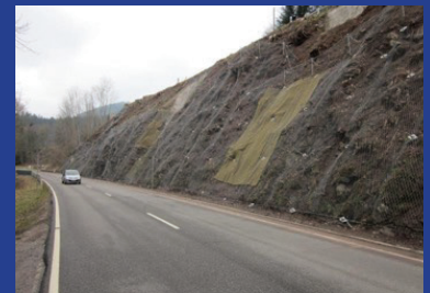
Example of Slope Stabilization in Progress
