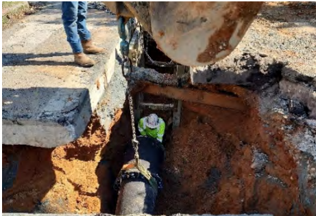
7 th St. & Constitution Ave. 20" Ductile Iron Pipe Install
