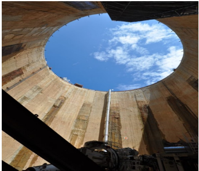
Clean Rivers Tunnel Construction Shaft
