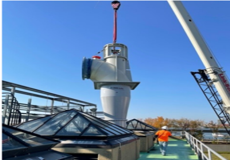
Blue Plains Filter Influent Pump Install
