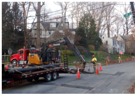
Small Diameter Water Main Rehab
