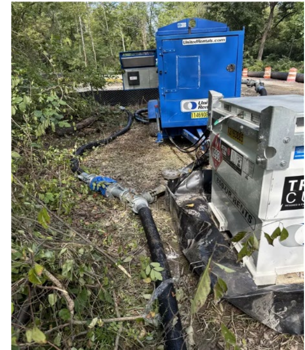
Push pit excavation and installation of wellpoints showing groundwater-control work.
