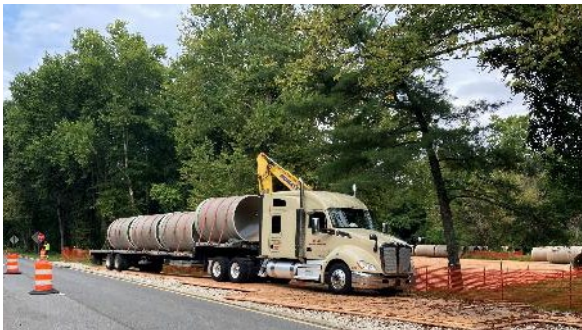
72-in pipe delivery start
