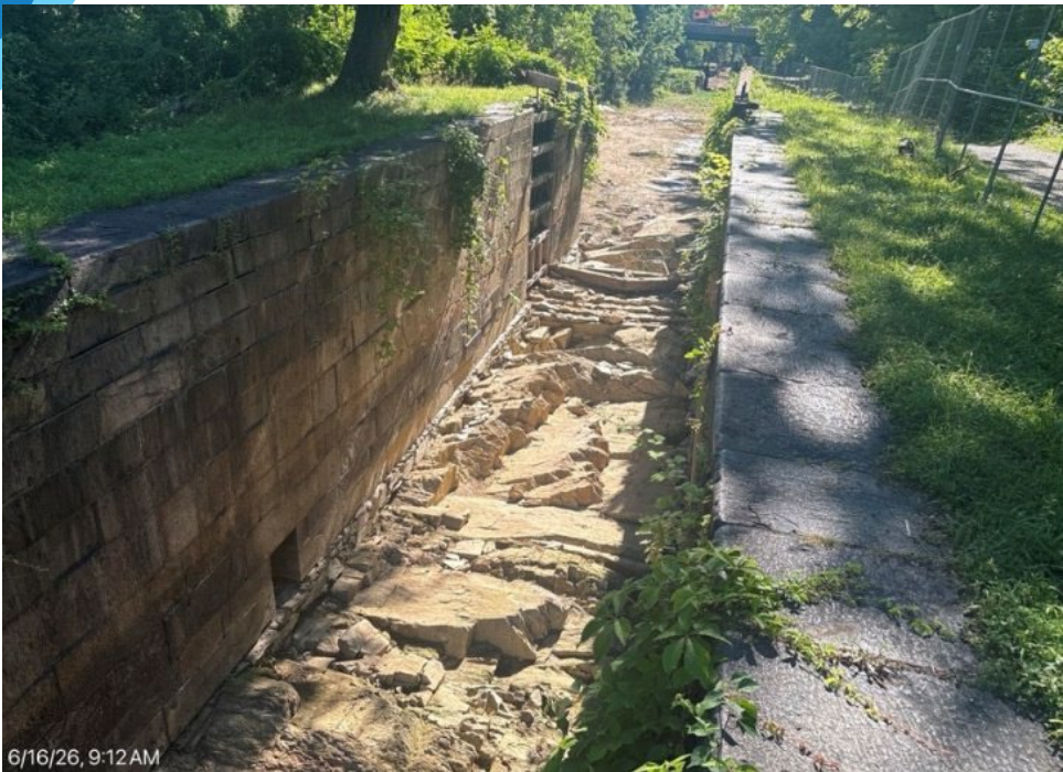
Lock 14 (Area 4) Cleaned to Bedrock
