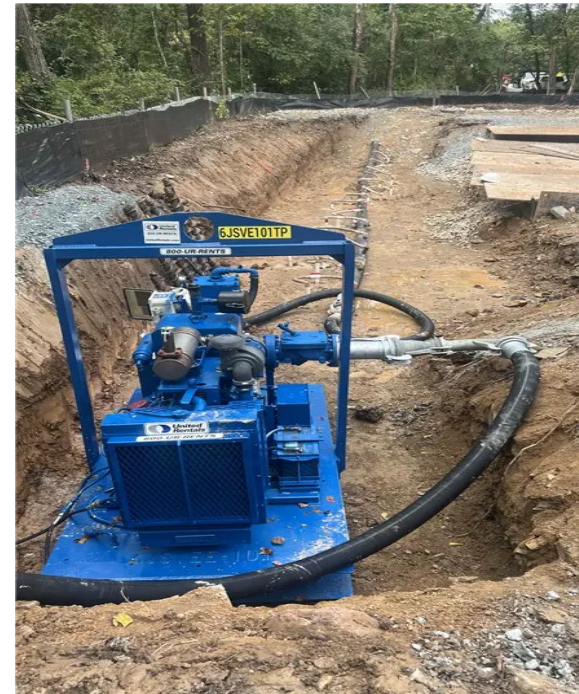
Push pit excavation and installation of wellpoints showing groundwater-control work.
