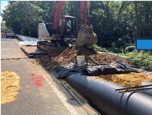
Bypass trench building, 5 th location (before)
