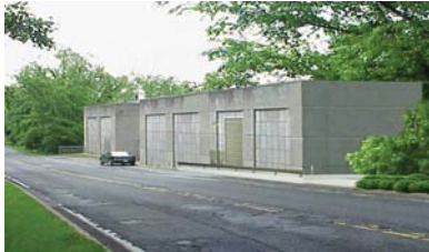
Site 4 – Little Falls Pumping Station Bethesda, MD
