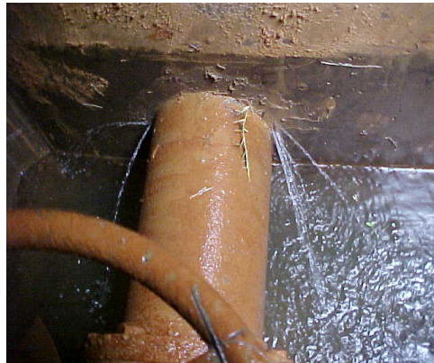
Meter Support Deficiencies
