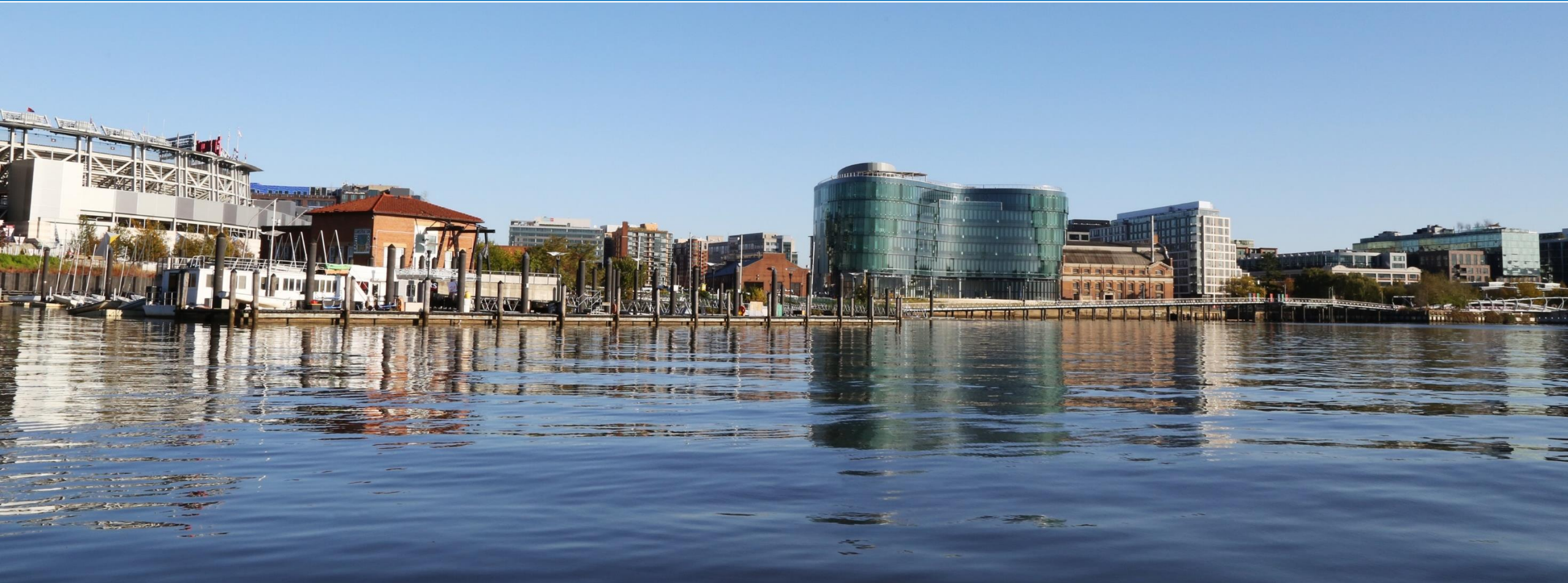
DC Water Headquarters from the Anacostia River
