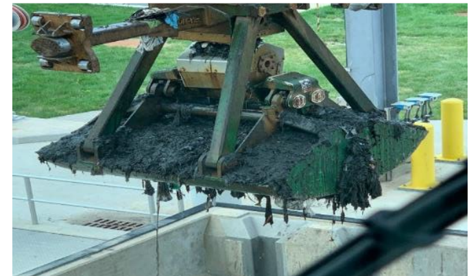
Trash, Debris and Solids Removal from Screening Shaft at Tunnel Dewatering Pumping Station
