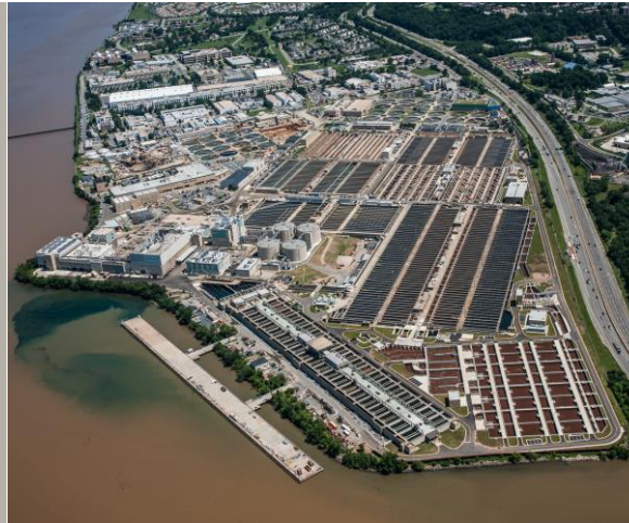
Blue Plains Advanced Wastewater Treatment Plant
