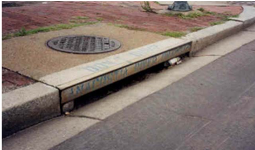
City Street Catch Basin
