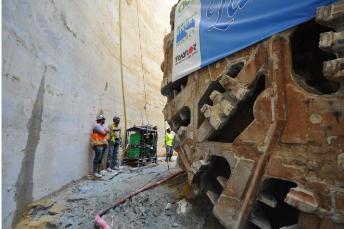
Blue Plains Tunnel Boring Machine, Ladybird
