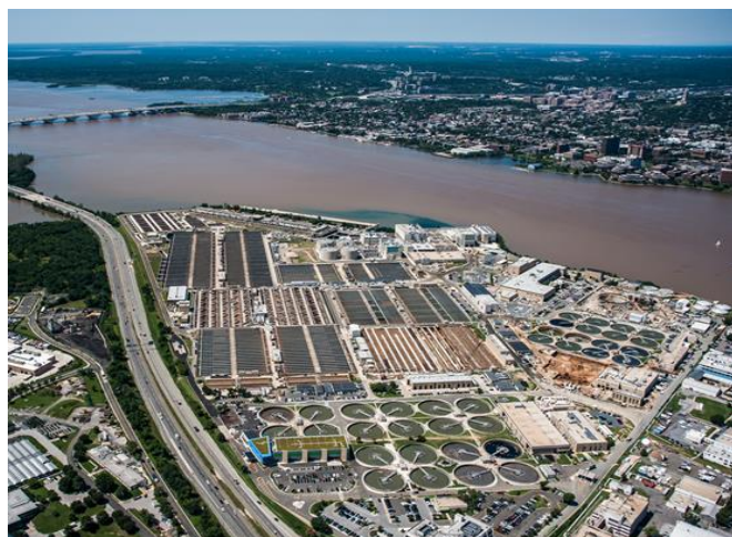
Blue Plains Advanced Wastewater Treatment Plant
