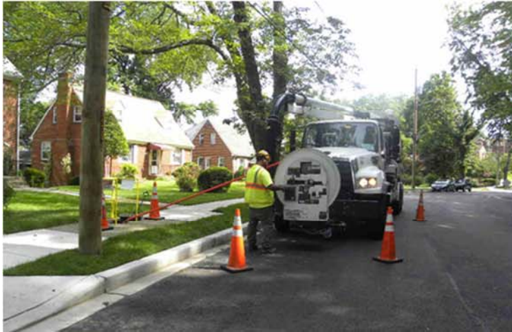
Work on Sewer Laterals
