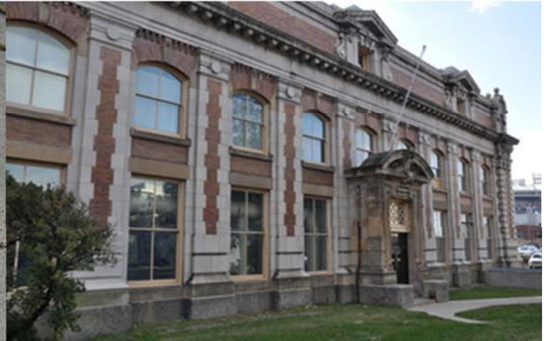
Main Pumping Station
