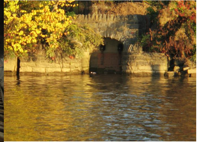
Combined Sewer Overflow Outfall
