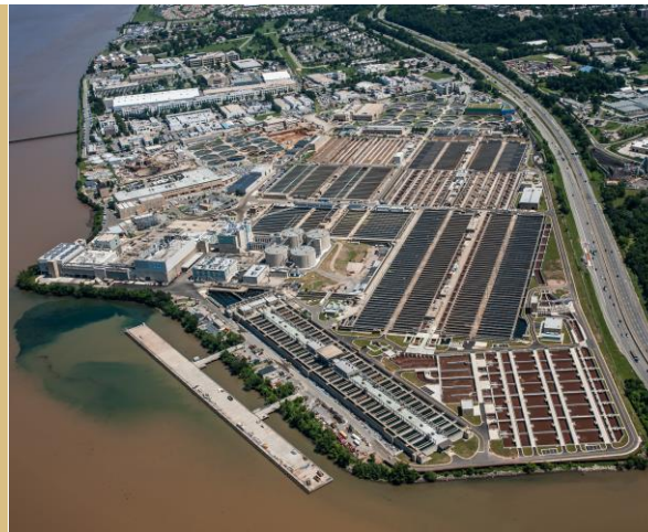
Blue Plains Advanced Wastewater Treatment Plant
