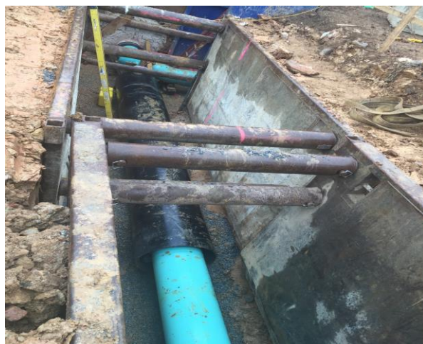
Work on Sewer Laterals
