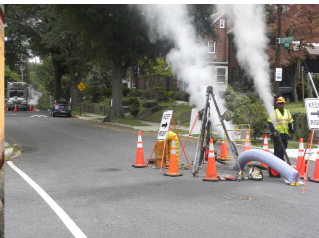
Sewer Rehabilitation - CIPP
