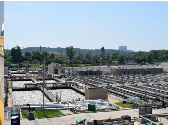
Nitrification Reactors
