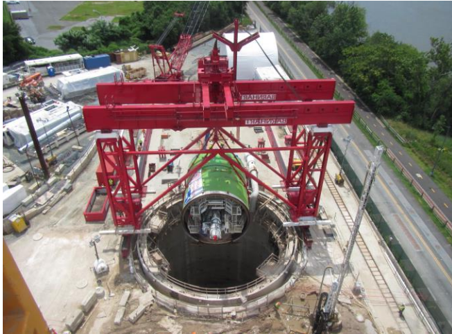
Anacostia River Tunnel Boring Machine, Nannie
