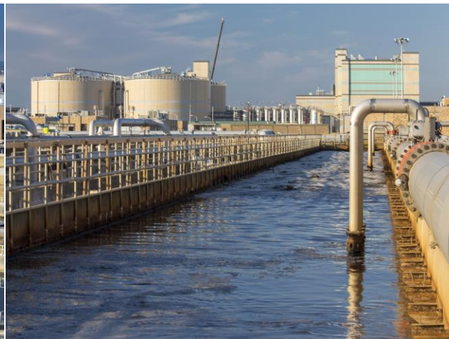
Secondary Sedimentation
