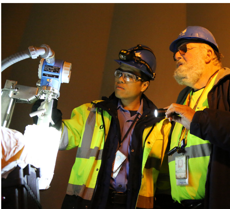
Anacostia Pumping Station inspection
