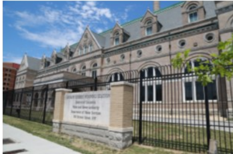
Bryant Street Pump Station
