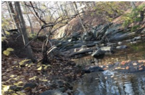
Sewer Rehab Soapstone Valley Park
