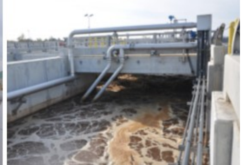
Nitrification Reactors
