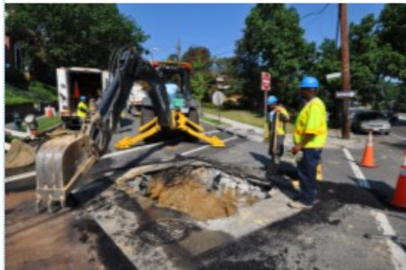
Sink Hole Rehabilitation
