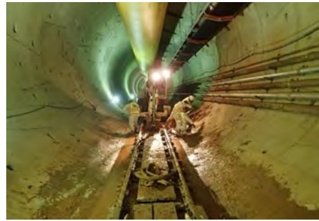
Northeast Boundary Tunnel
