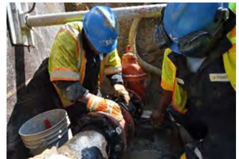
Water Meter Installation
