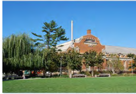
Main Pumping Station
