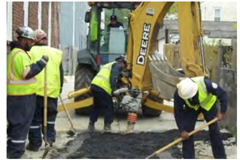
Linear Pipe Restoration
