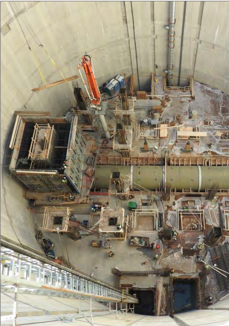
Clean Rivers Tunnel Dewatering Pump Station
