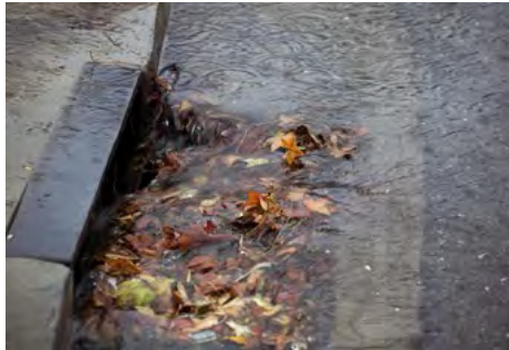
City Street Catch Basin
