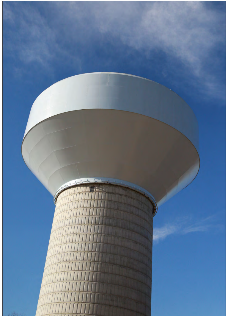
Saint Elizabeth Water Tower
