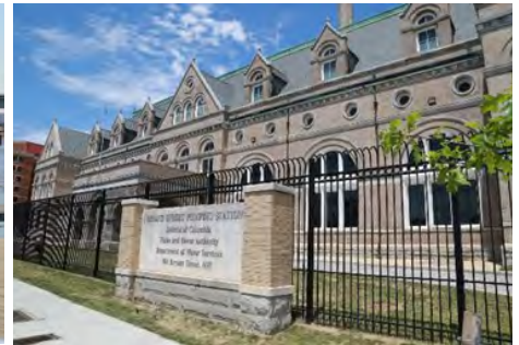
Bryant Street Pump Station
