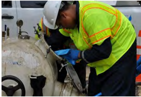
Sewer Line Rehabilitation Perma-liner
