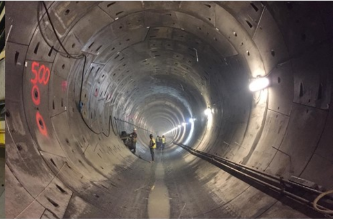
Combined Sewer Overflow
