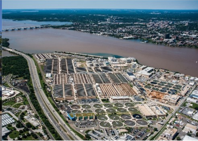
Blue Plains Advanced Wastewater Treatment Plant
