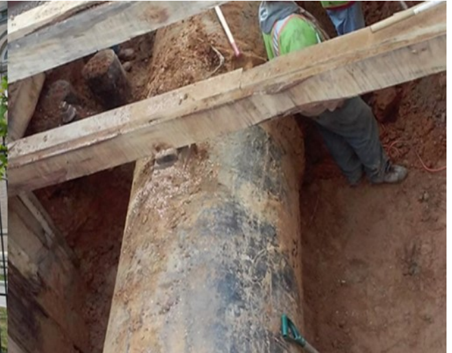
Large Valve Replacement
