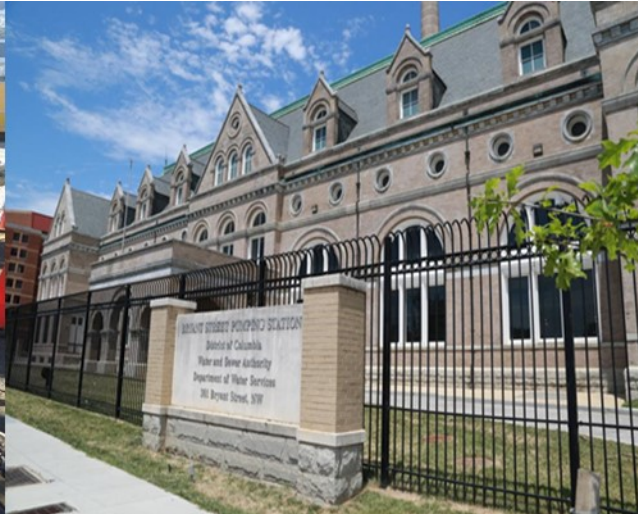
Bryant Street Pumping Station
