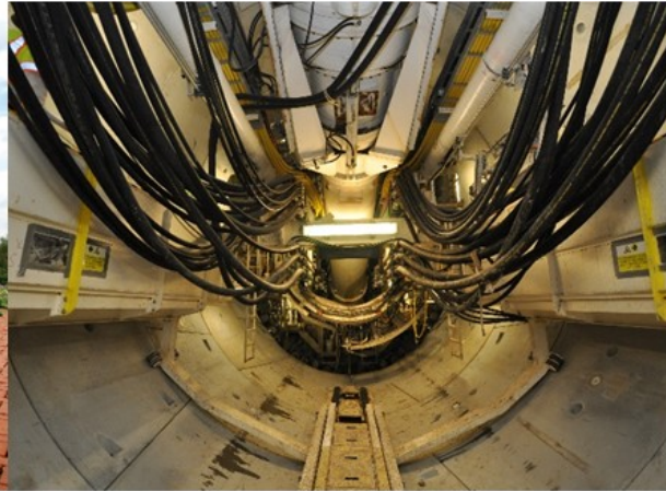
Tunnel Boring Machine
