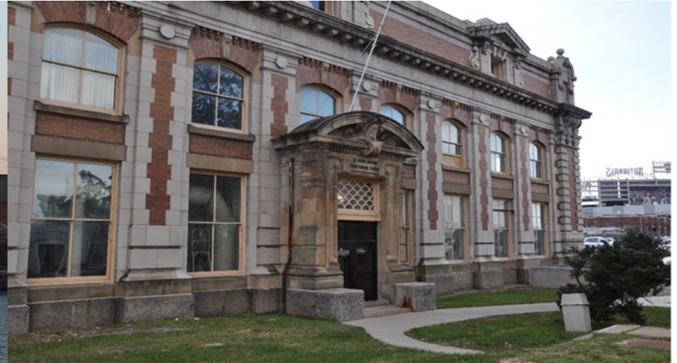
Main Pumping Station
