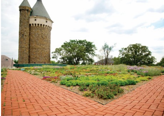
Fort Reno Green Roof
