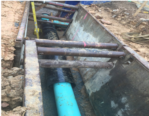
Work on Sewer Laterals
