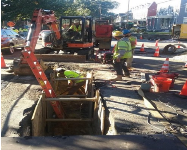
Small Diameter Water Main Replacement
