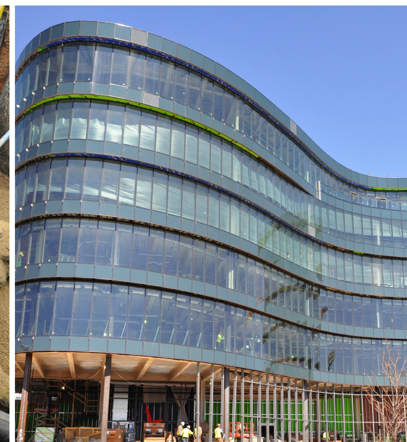
New Administrative Building Under Construction on SE Waterfront
