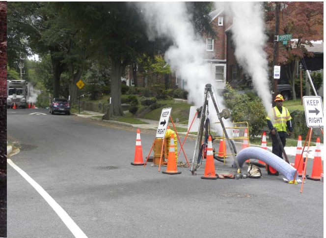
Sewer Rehabilitation - Cured In Place Pipe Lining (CIPP)
