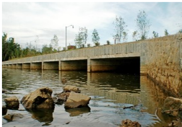
CSO 19 Overflow Facility
