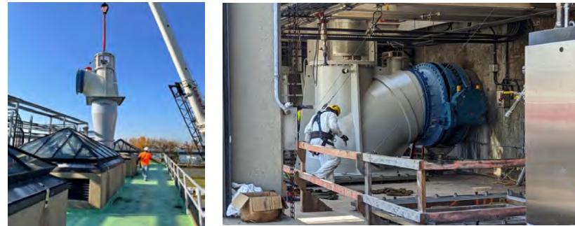
Filter Influent Pump 1-10 Replacement Project
