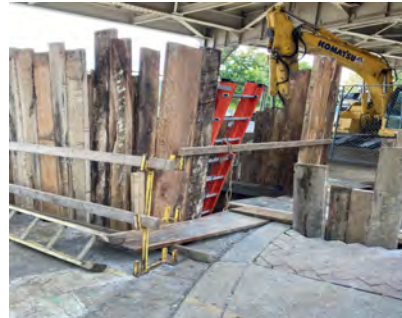
Shoring at K St NW
