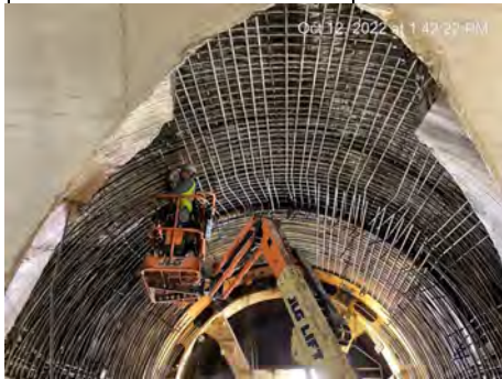
FSCT Second CIP Lift Reinforcement NEBT Sawcutting FLA Adit Shotcrete
