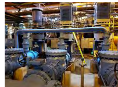
Reclaimed Final Effluent Pump Station Upgrades
