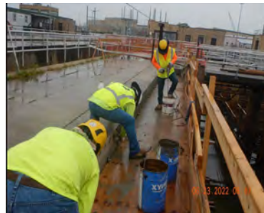
Sedimentation Basin 12 Concrete Repairs
