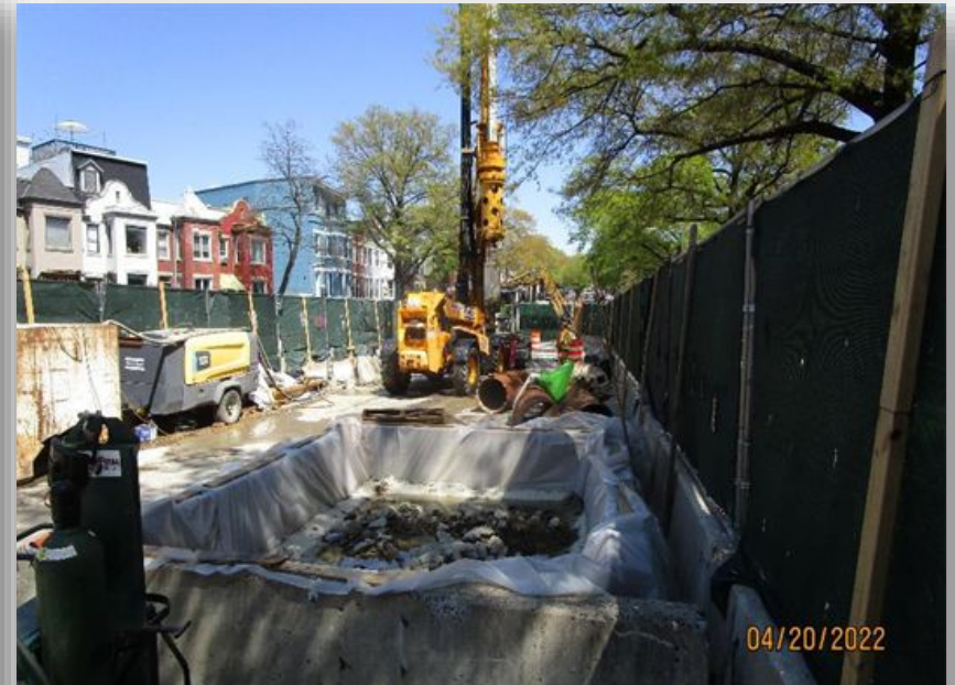
Junction Manhole Construction
