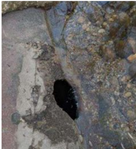
Sewer break with creek water infiltration in Soapstone Park (2020)
