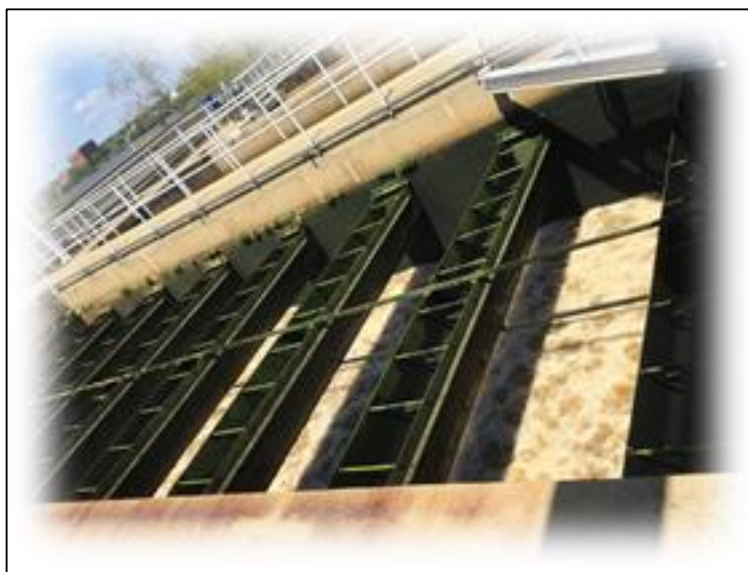
Figure 1. Normal filter backwash cycle showing submerged underdrain.
