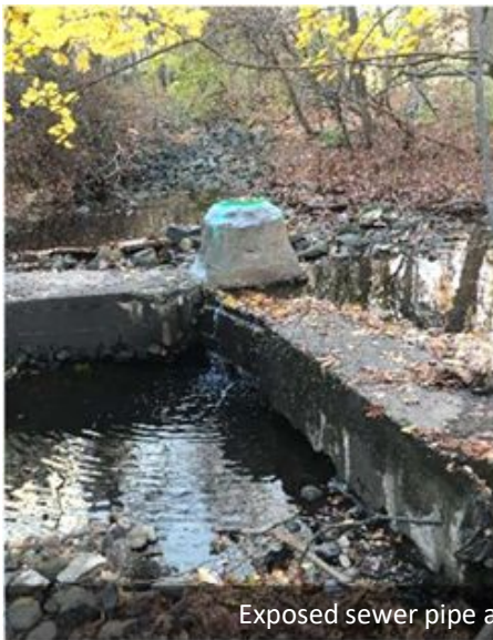
Sewer break with creek water infiltration in Soapstone Park (2020)
