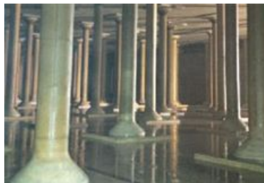
Third High Reservoir
