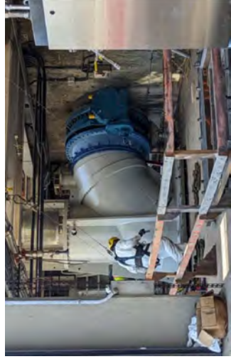
Filter Influent Pumps 1-10 Replacement Project
