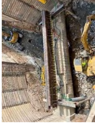
Potomac Interceptor @ MH31: Pipe Support
