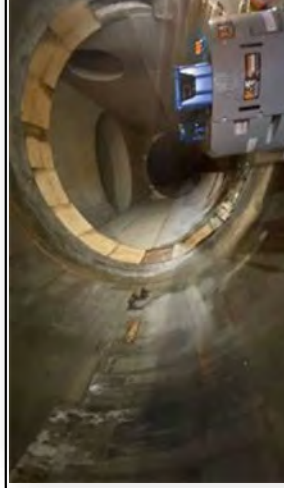
Tunnel Bulkhead removed at CSO 019
