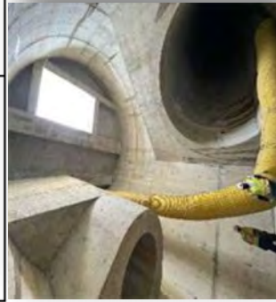
R Street Shaft
