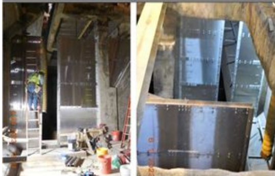
Grit Chamber Baffle Wall Project
