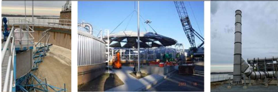
Gravity Thickener Upgrades GT-1 through GT-10
