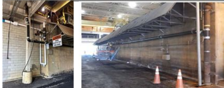
DSLFL Safety Repairs
