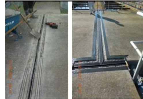
Nitrification Sedimentation Expansion Joints Repair
