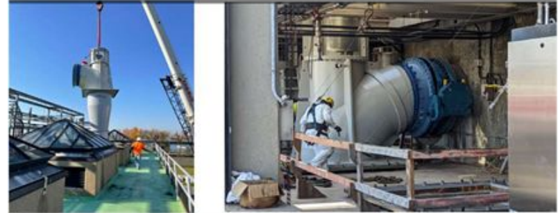
Filter Influent Pumps 1-10 Replacement Project
