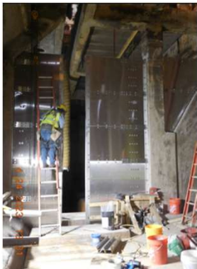
Grit Chamber Baffle Wall Project
