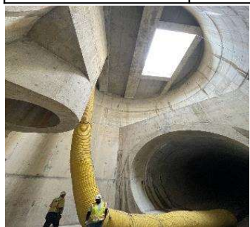
R Street Shaft
