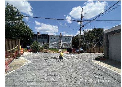
Alley Permeable Pavement (APP 36-08 A/B)
