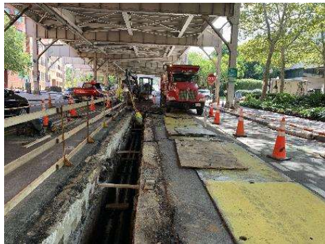
Trench Relocation at CSO 024
