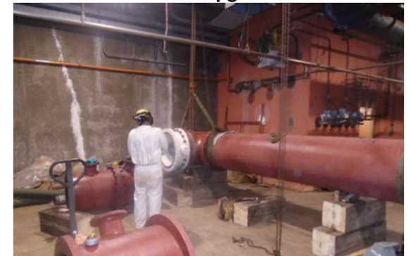
Reclaimed Final Effluent Pump Station Upgrades
