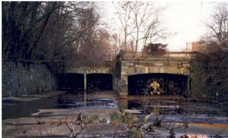
CSO 049 in Dry Weather
