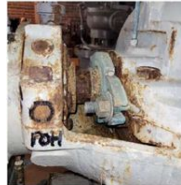
Figure C.25: Pump Packing, Typical
