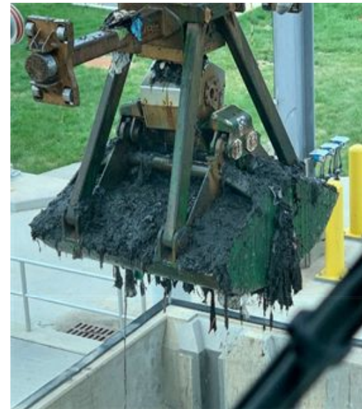
Trash, Debris and Solids Removal from Screening Shaft at Tunnel Dewatering Pumping Station
