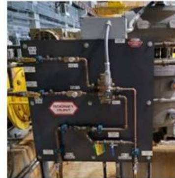
Figure C.13: Cone Valve – Typical Control Panel
