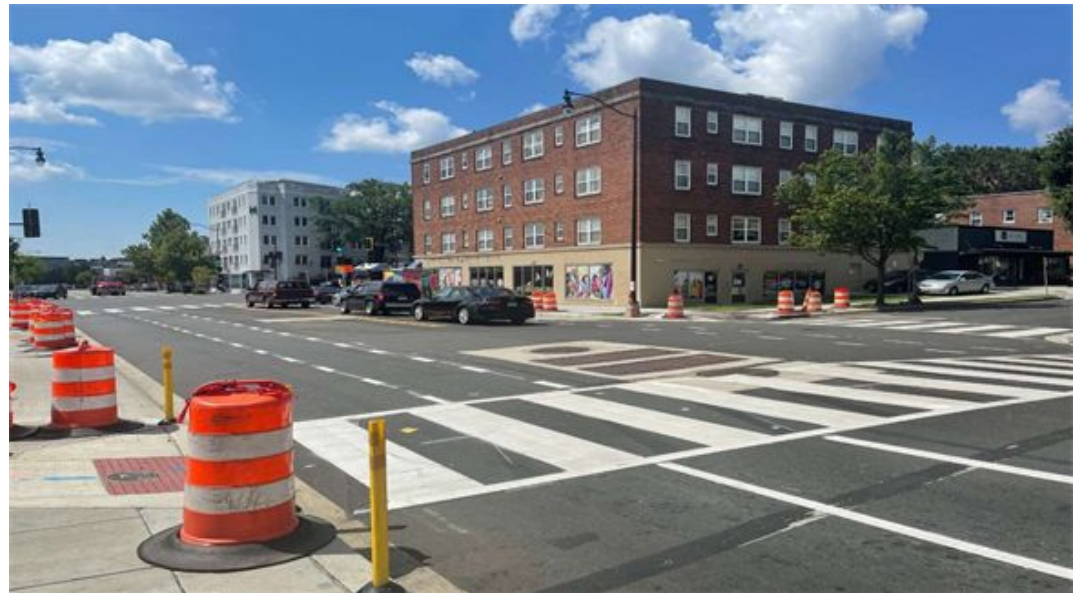
4 th Street Restoration
