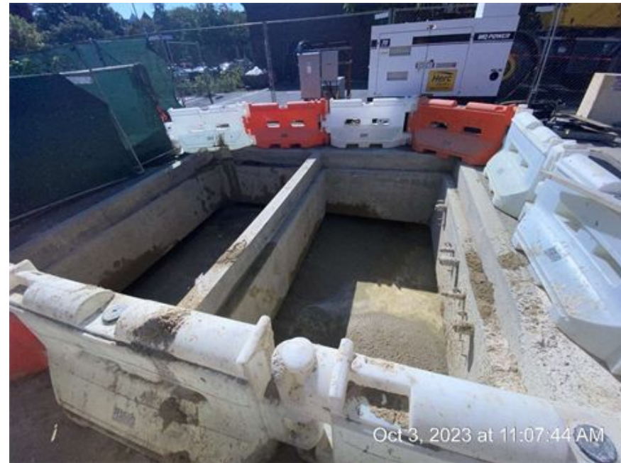
Pump Station Shaft
