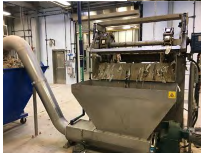
Poplar Point Pump Station
