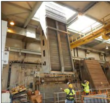
Replacing/Upgrading Influent Screens
