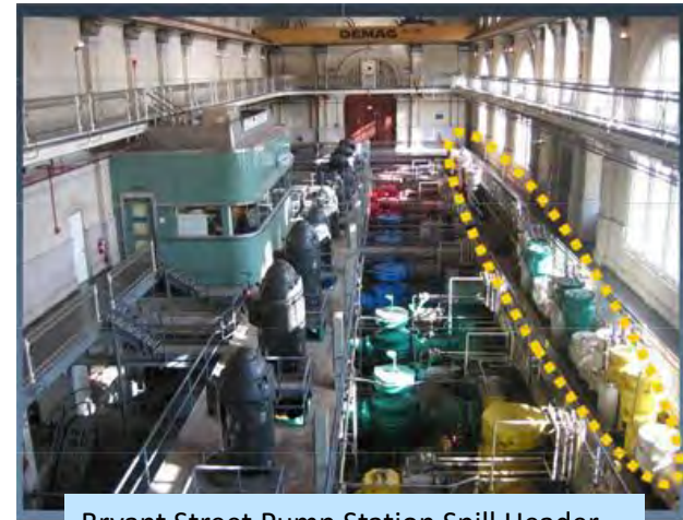
Bryant Street Pump Station Spill Header
