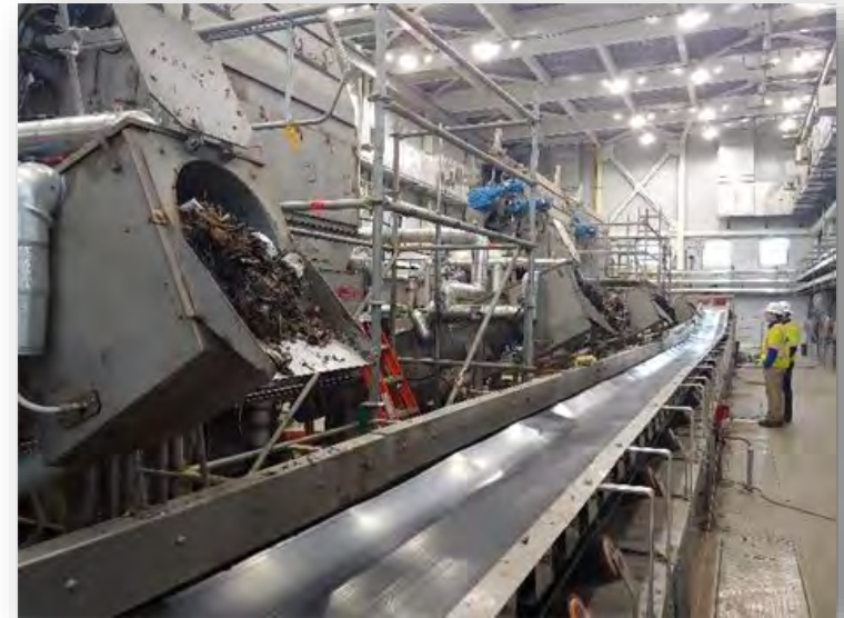
Anacostia Tunnel from Mar 2018 – Dec 2022:
